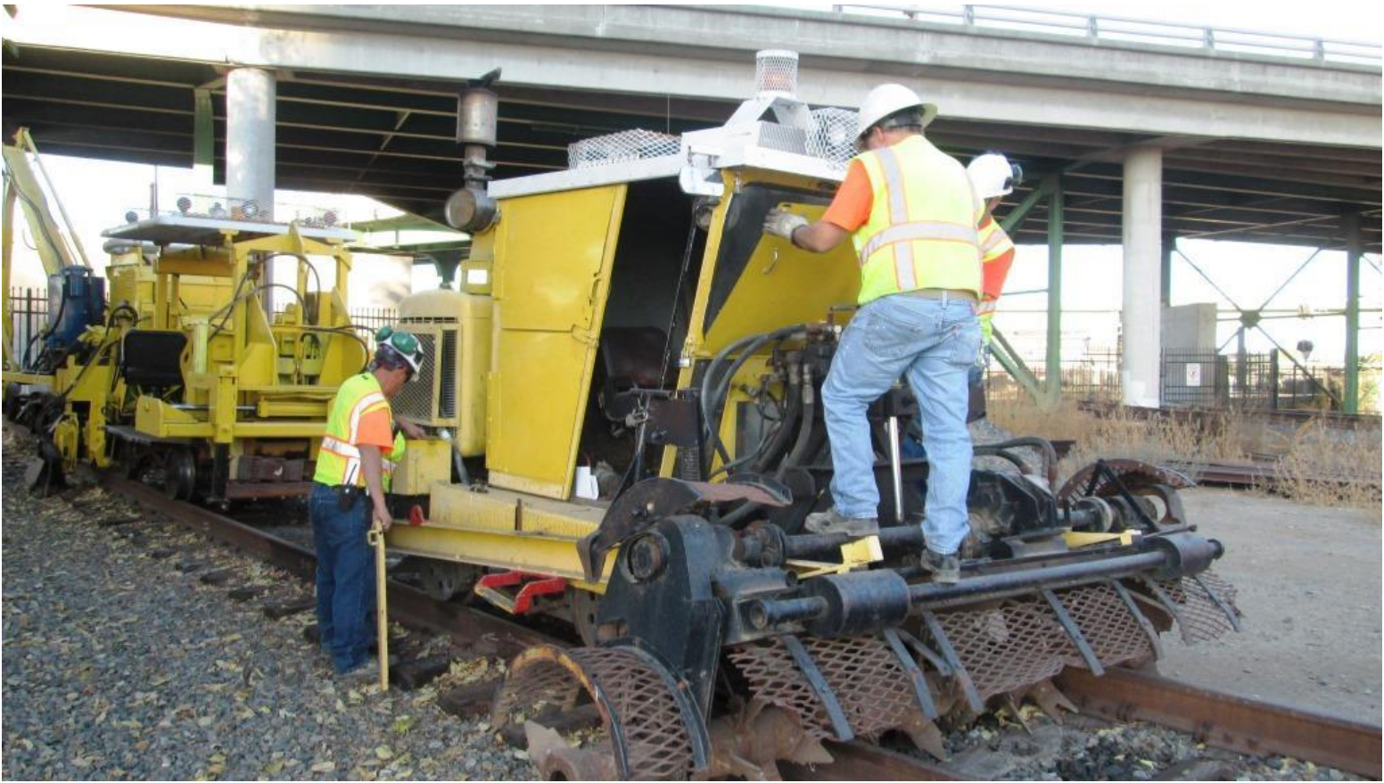
Joe, Mike H., and Ed get the scarifier-inserter opened-up
