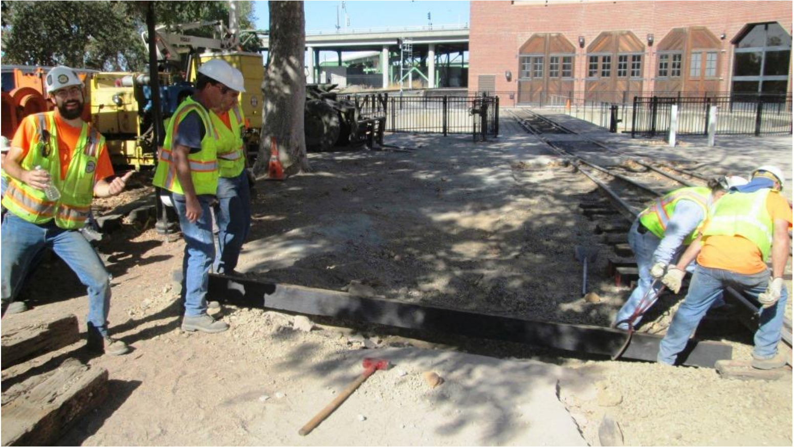
Matt "photo-bombs" the moment Heather and Mike M. drag the 14-foot switch tie under the base of the rail...
