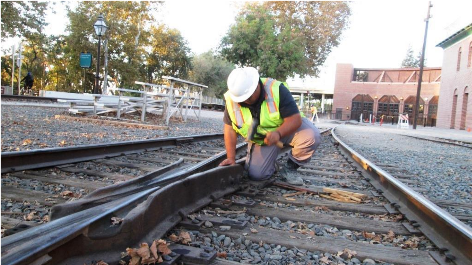
Anthony spikes down the wayward plates at the Switch 2 frog
