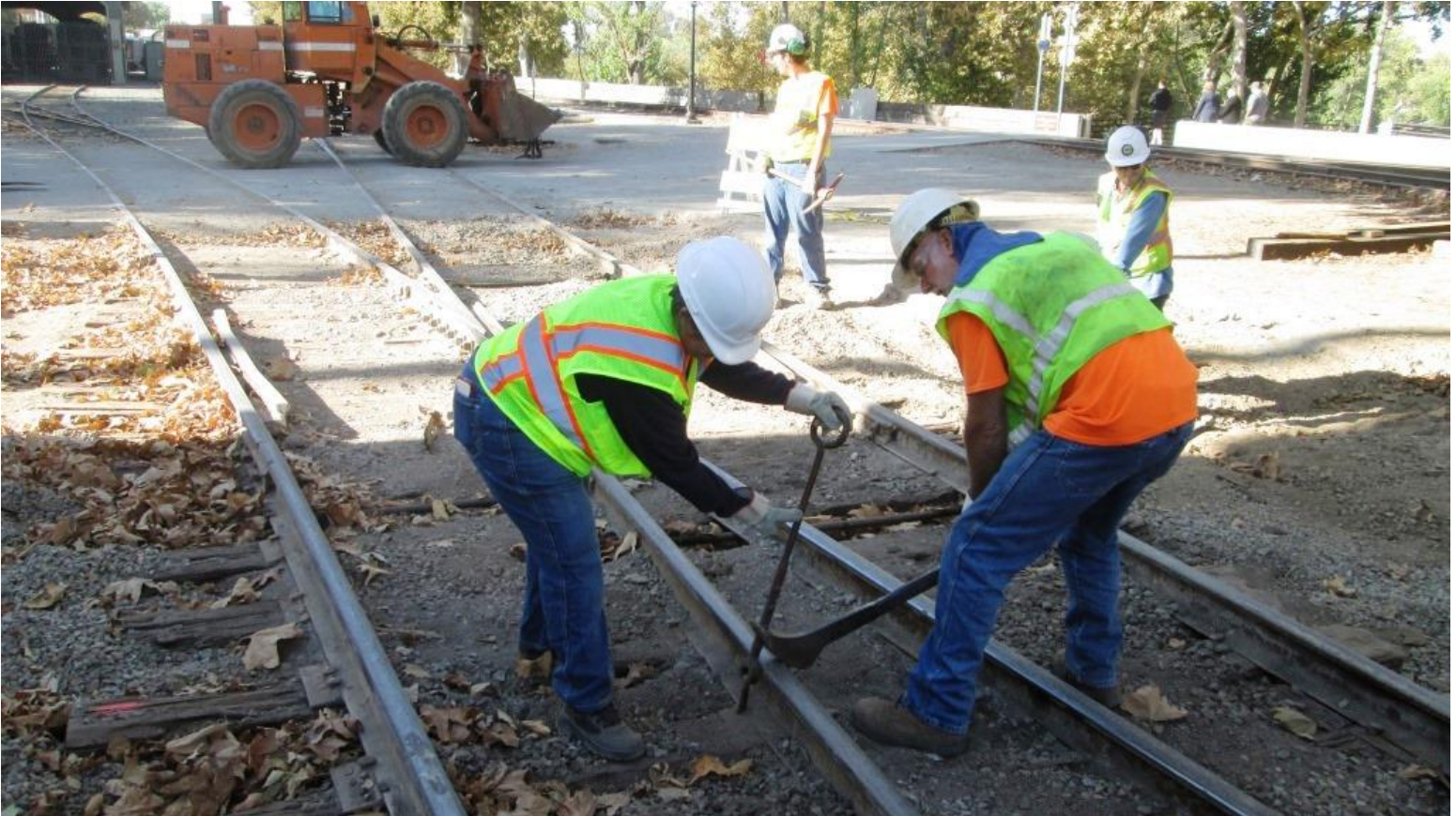
Pam uses the "road-master" to grab the spike while Mike M. pulls it with a claw-bar
