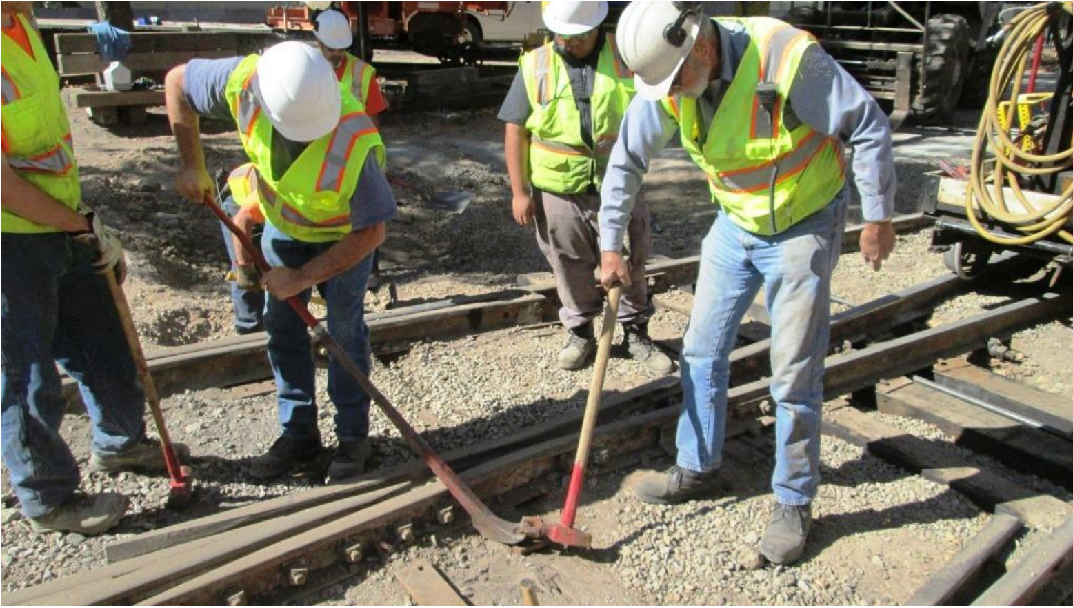
Andrew is able to get the claw-bar beneath the spike-lifter
