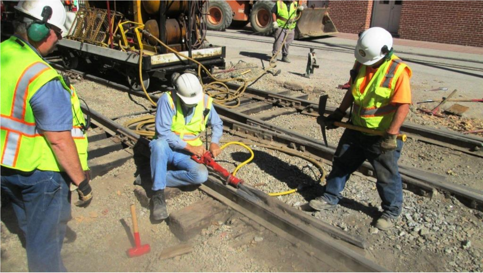
Alan uses the chipping hammer to break-up concrete and compacted dirt between the guard-rail and stock-rail
