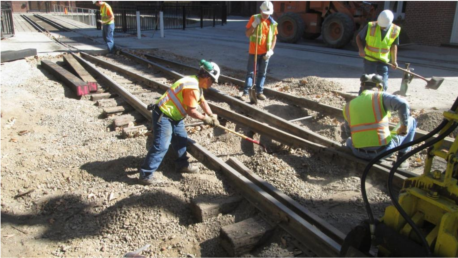
Joe, Mike M., Andrew, and Alan act as human scarifiers...
