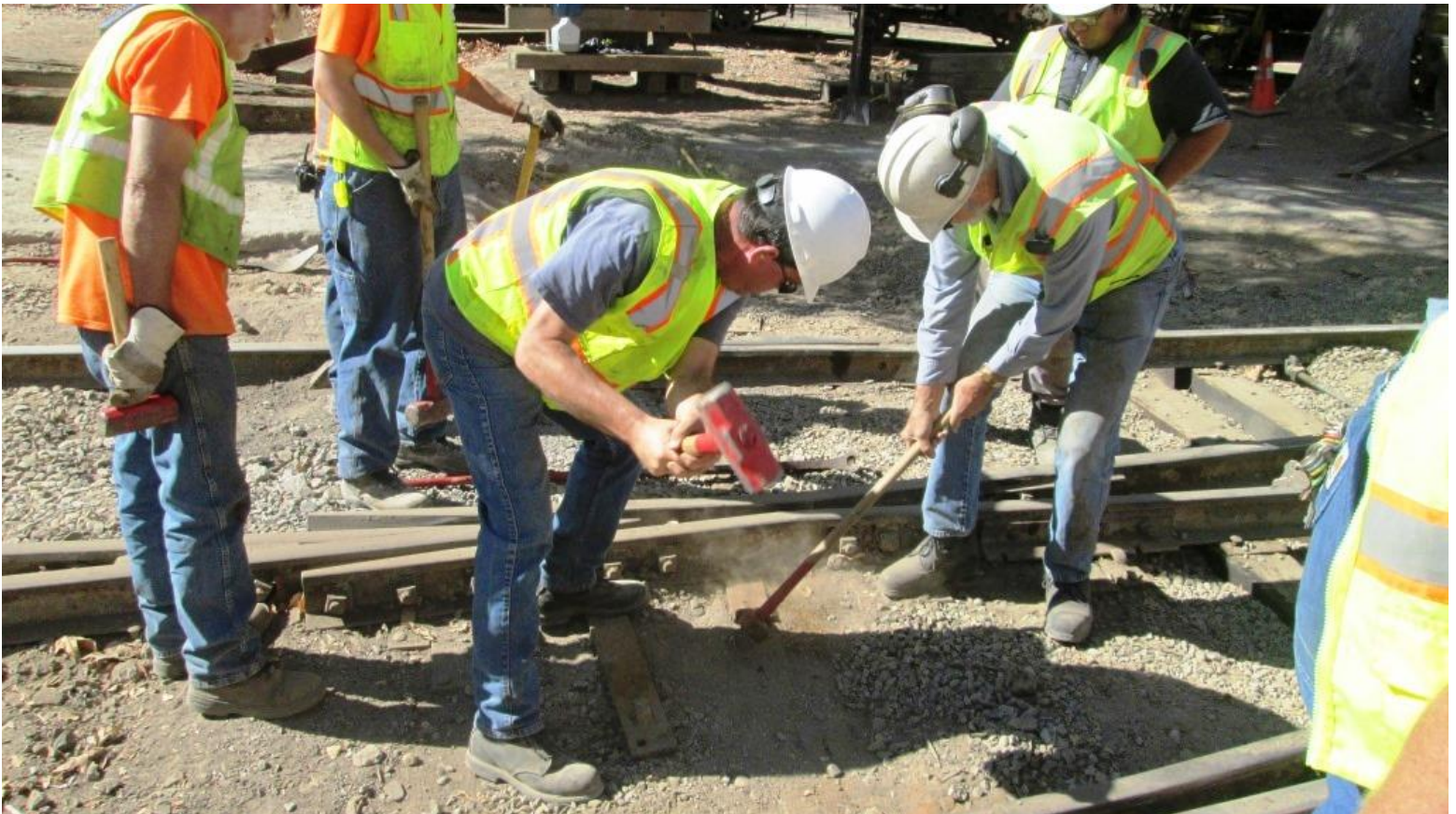
Andrew and Alan employ the spike-lifter to pry-up another corrosion-fused spike from a frog-plate
