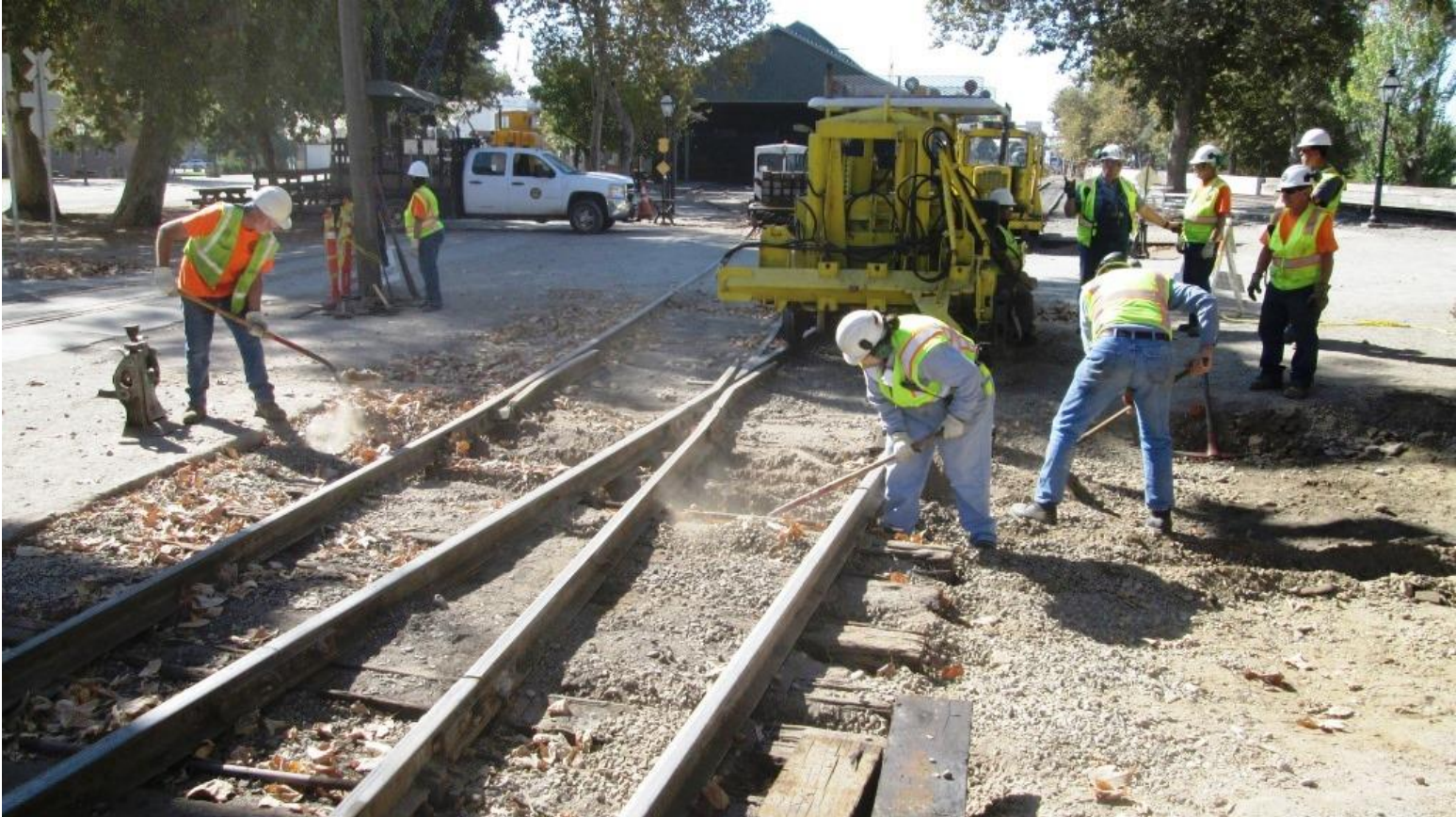
With all the converging rails, the scarifier won't work so Mike M., Heather, and Alan dig out the tie-cribs by hand
