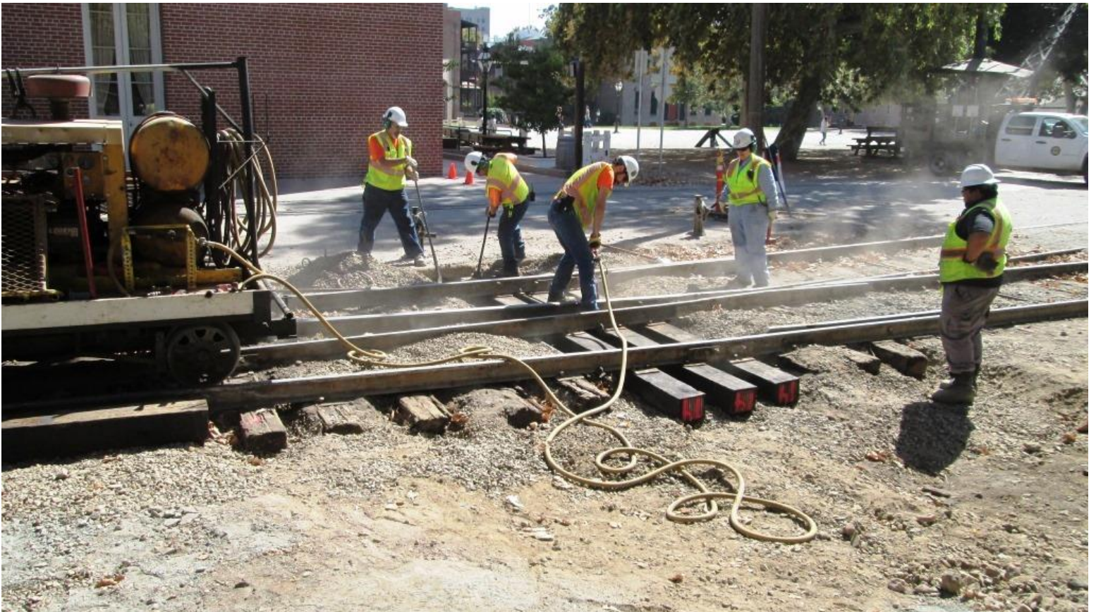
Ed and Joe nip-up the tie as Matt drives the spikes
