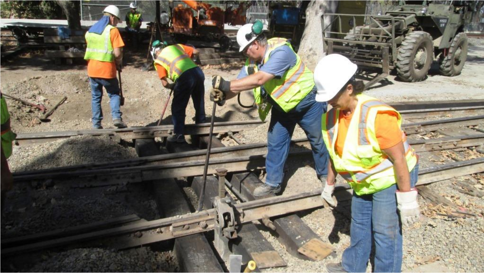
Mike M., Ed, Chris, and Pam shimmy the ties about to get them evenly spaced
