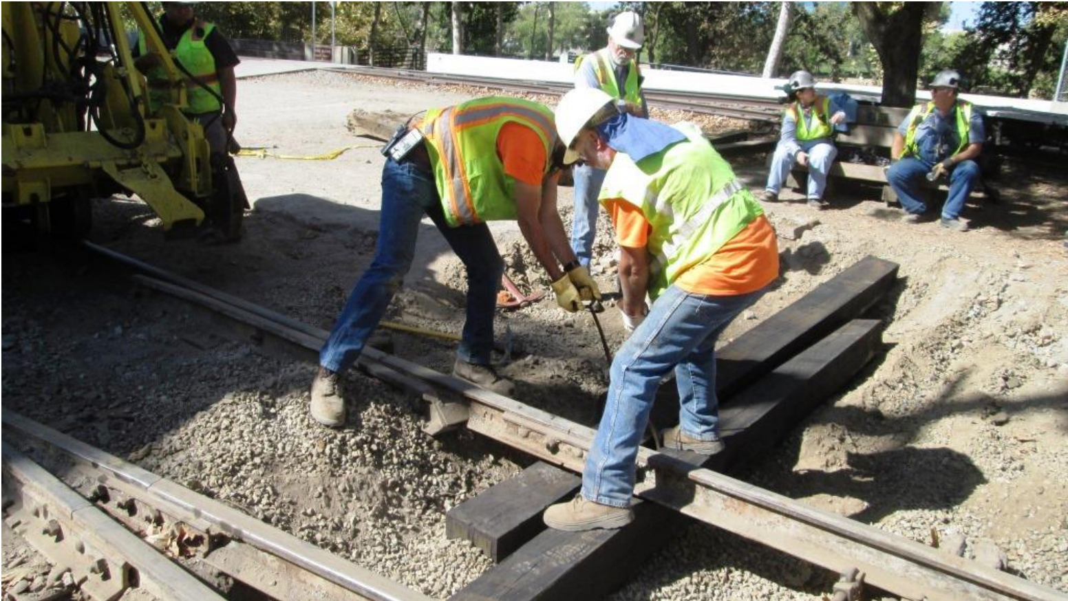
Matt and Mike M. drag a 14-foot hardwood tie into position
