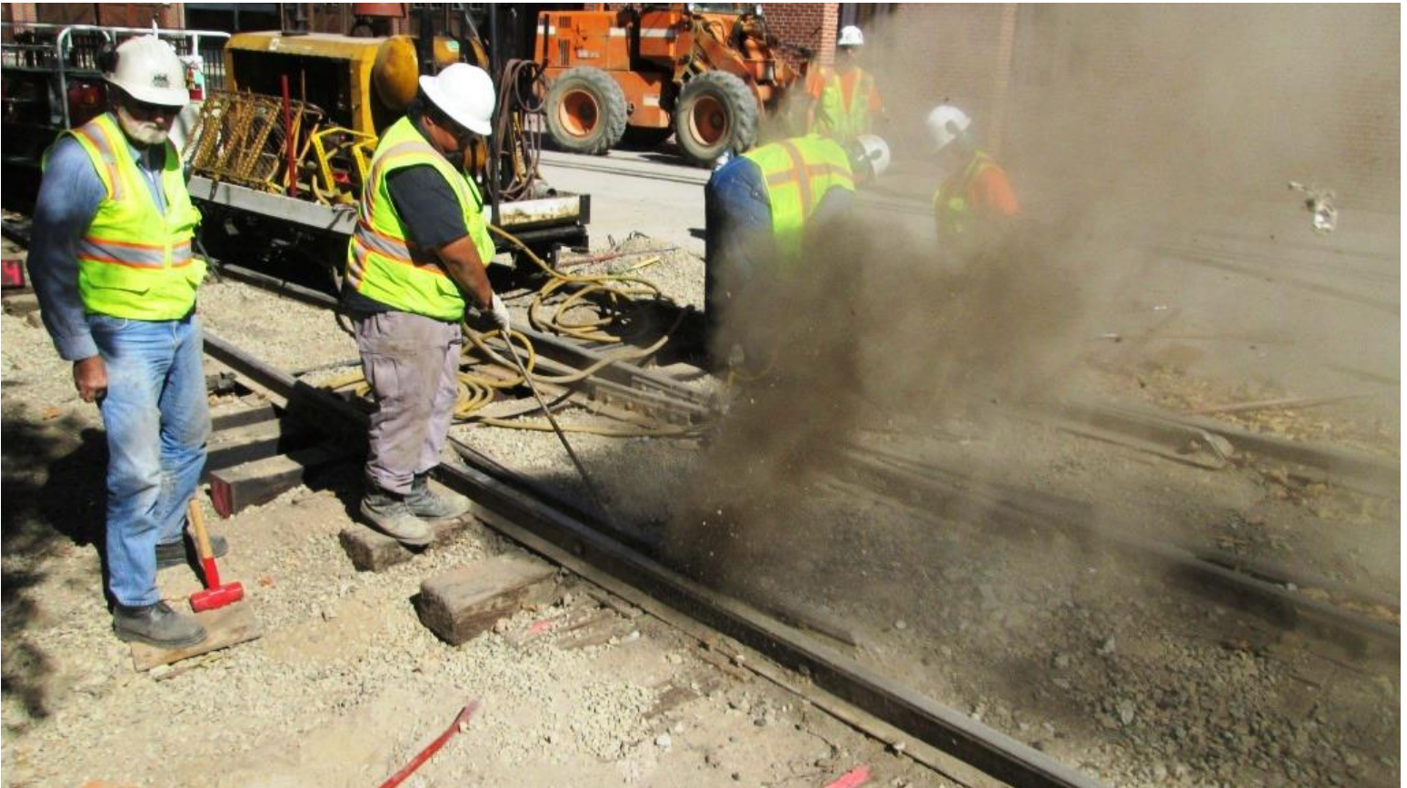
Anthony uses the air-wand to blast the debris from between the guard-rail and stock-rail
