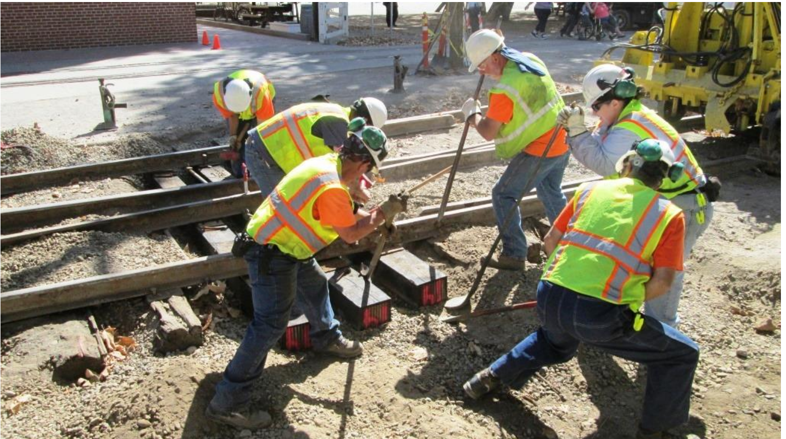
Weston and Andrew set spikes as Joe, Mike M., Heather, and Ed nip the ties up against the base of the rail
