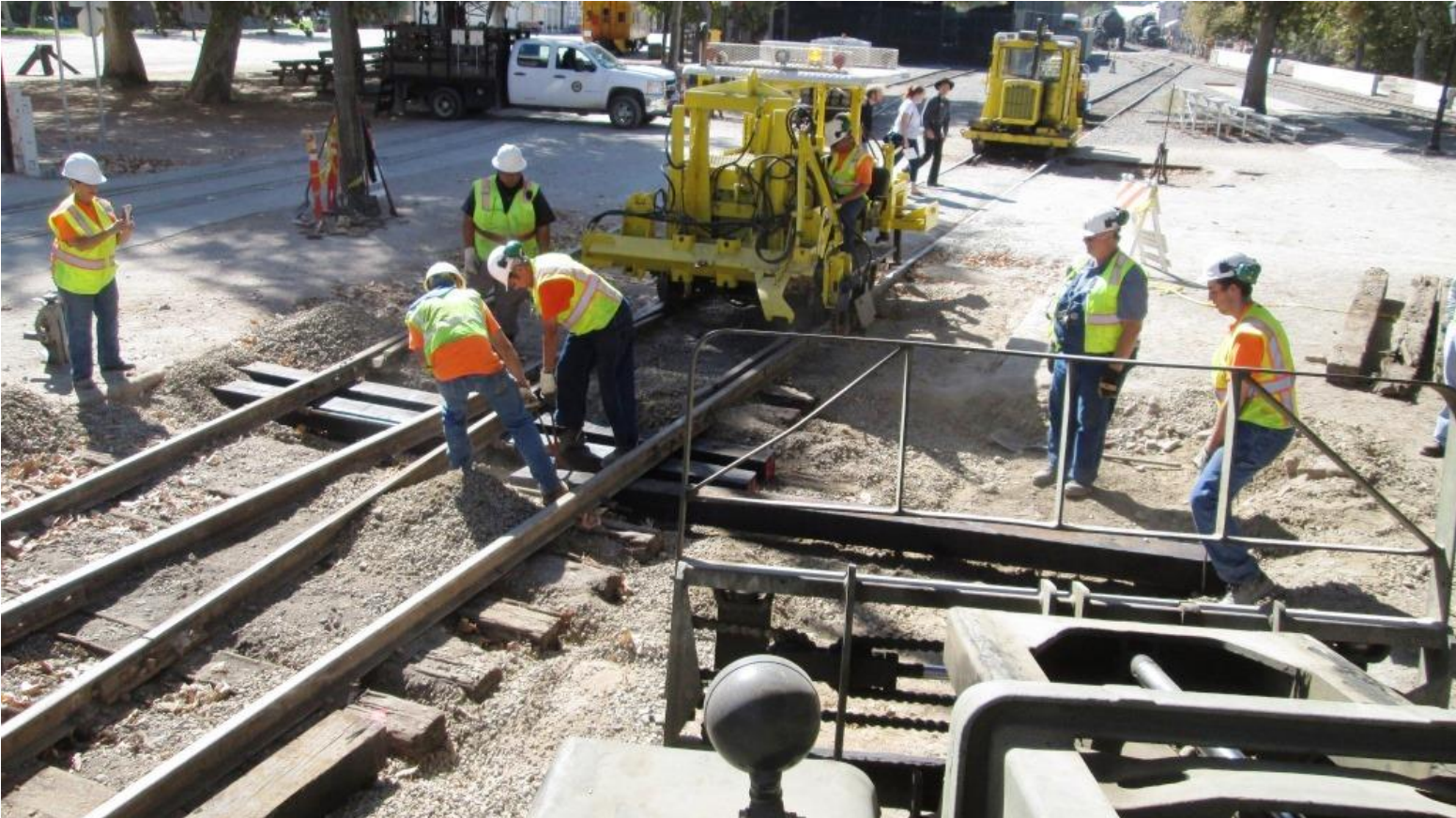
Mike M, Ed, and Weston move the next tie into position
