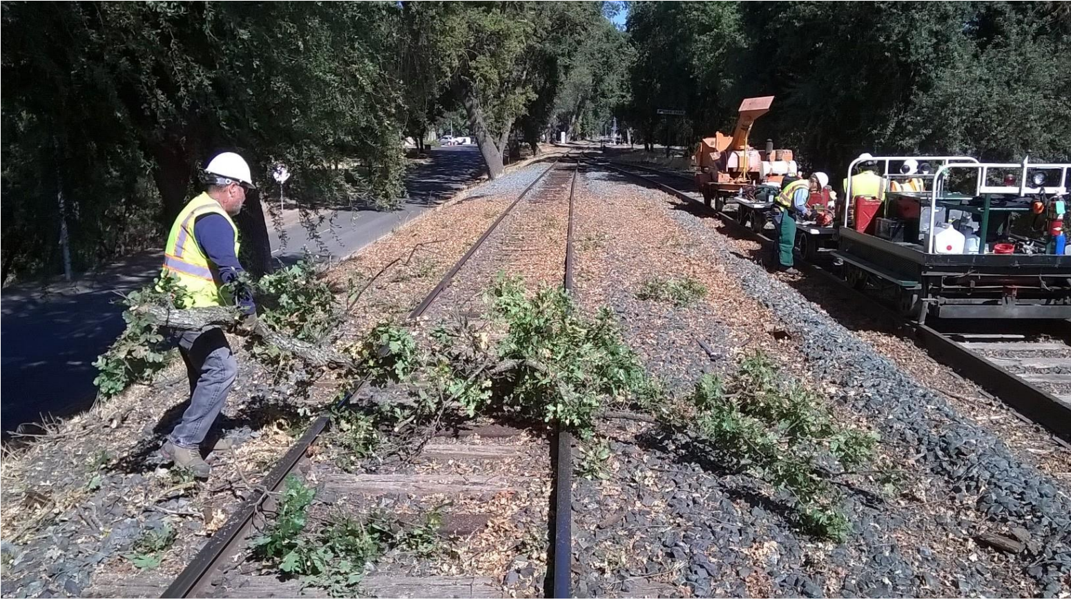
Steve moves oak debris for "compressing"
