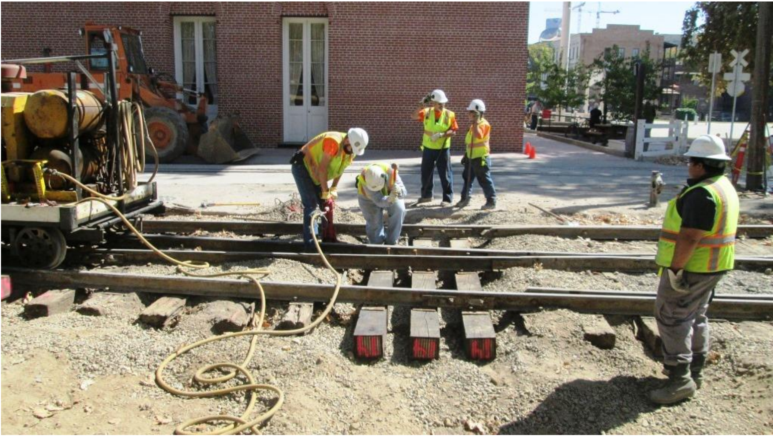
Heather sets a spike as Matt stands by to drive it down with the pneumatic spike driver
