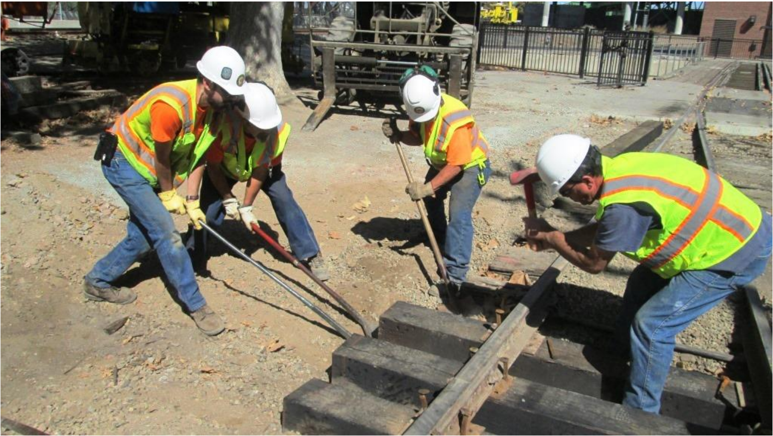
Matt and Ed nip-up the tie as Joe shoves rock beneath it while Andrews sets spikes
