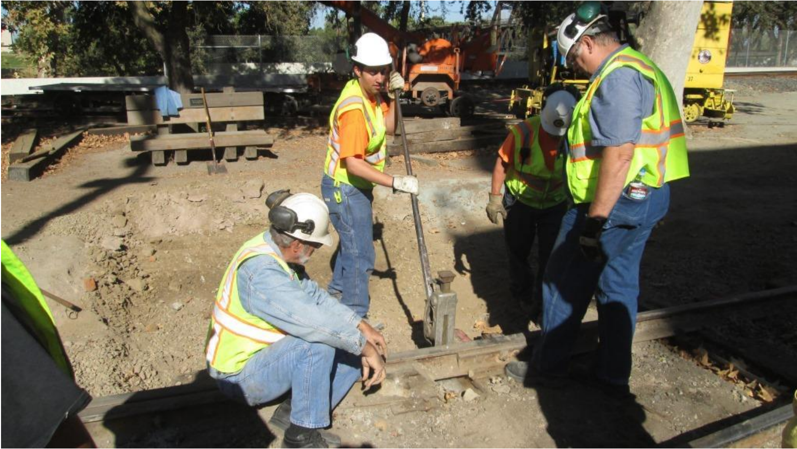
Weston cranks on the track-jack to relieve downward pressure on the tie
