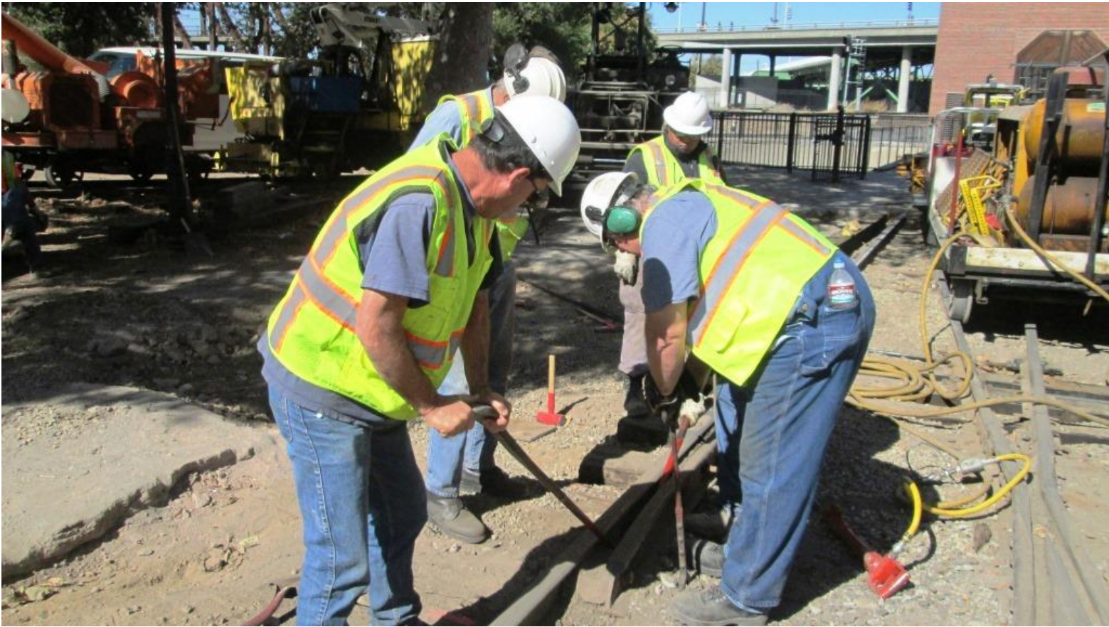
Andrew and Weston use the thin-ends of nippers and claw-bars to pry-up the spikes between the guard-rail and stock-rail
