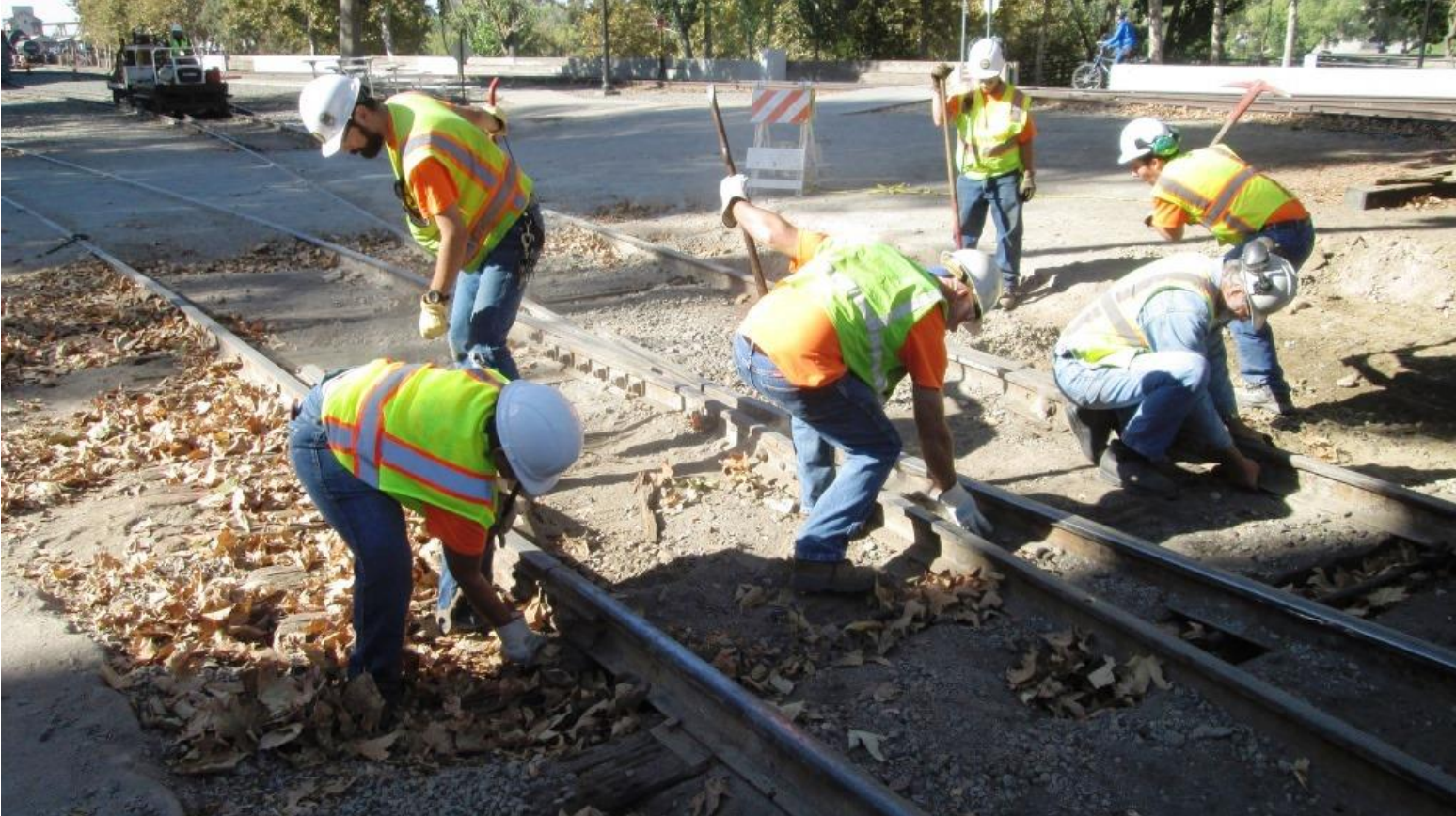
Pam, Matt, Mike M., Joe, Weston, and Alan all work to prepare ties for removal
