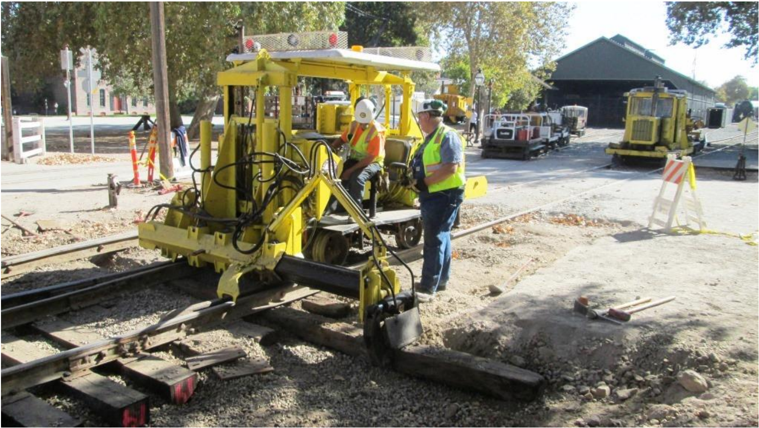
With the tie free of all spikes, Joe on the 125 pulls it out
